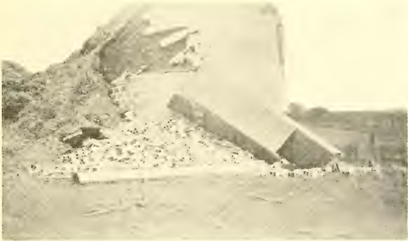
Forty-Two Acres of Corn Spoiled by the Collapse of This Clay Tile Silo
